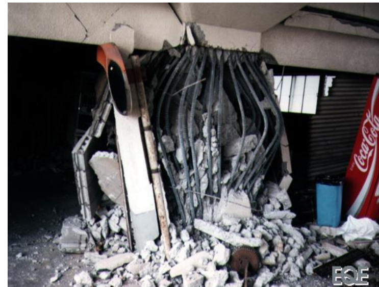
Poorly reinforced concrete
