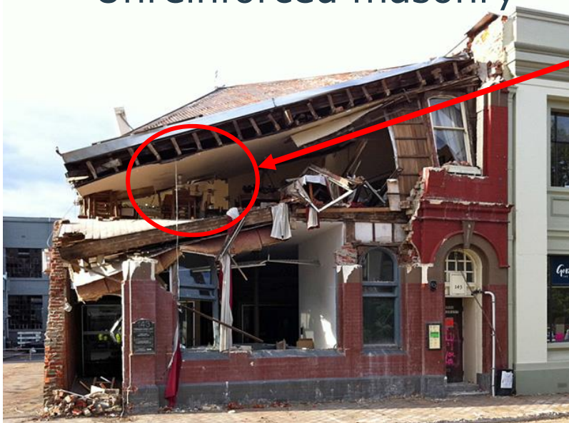
Unreinforced masonry
